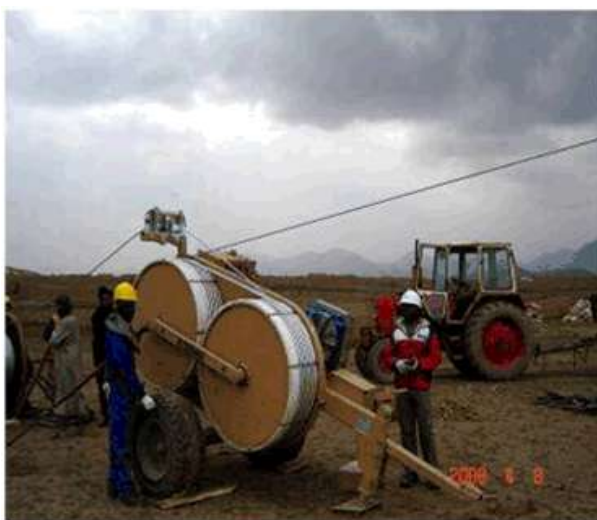
Picture 2: Transmission line construction - wiring
