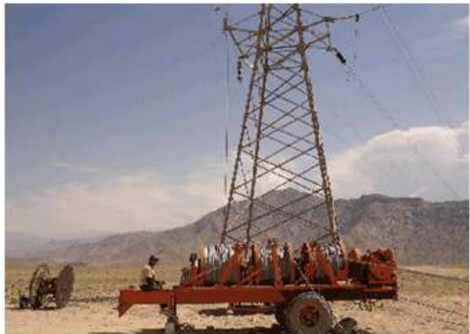
Picture 3: Construction in progress
