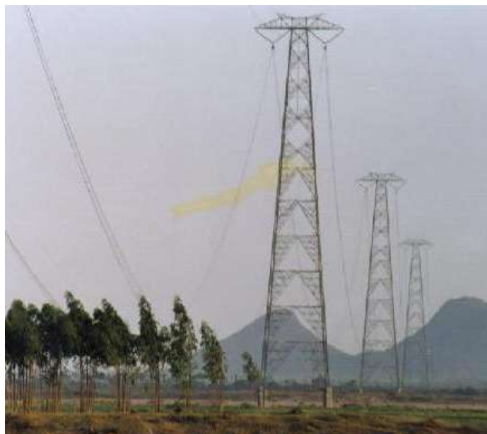
Picture 1: HVDC line after completion
