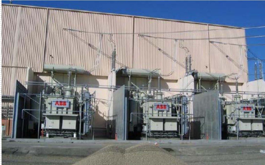
Converter Transformer
